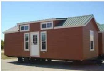
110 - Exterior with lap siding and metal roof
